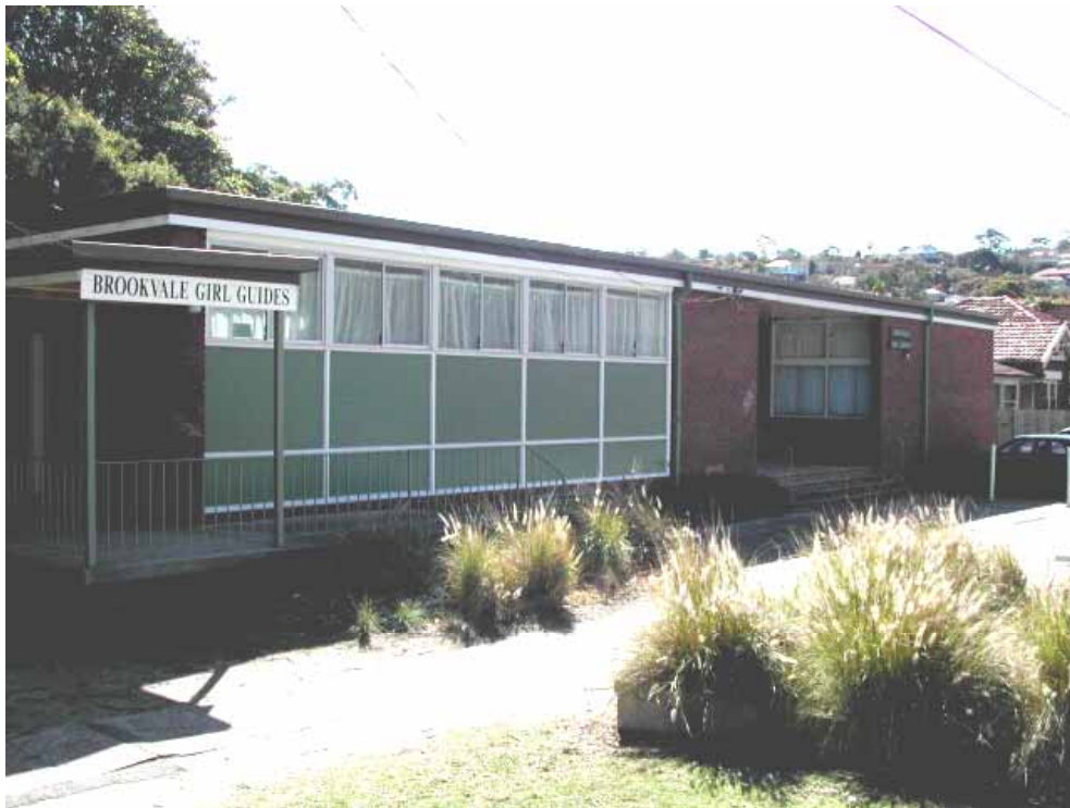
Figure 2. Existing building – Alfred Street façade
