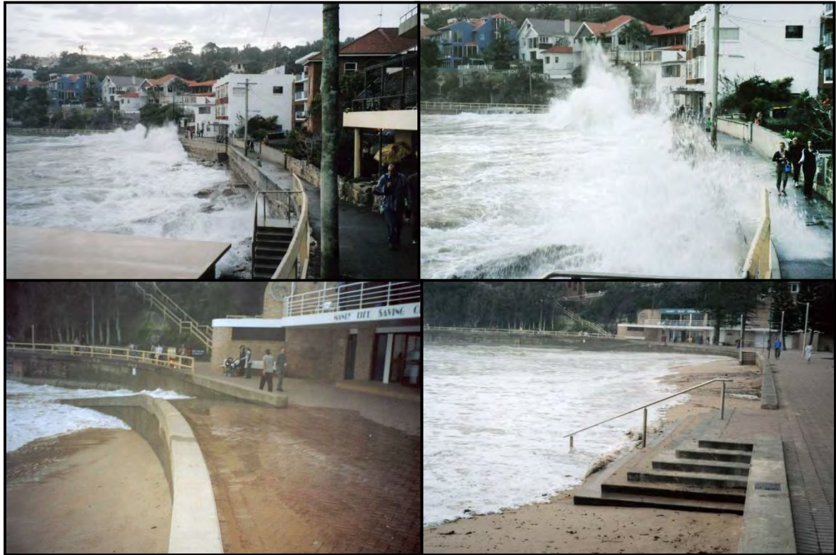
Figure 4.6 Top: Wave Overtopping at Fairy Bower; Bottom: Wave Runup at Manly LSC Boat Ramp and Manly Beach Stairs at Victoria Parade (26/06/2003. Photos James Carley, WRL)
