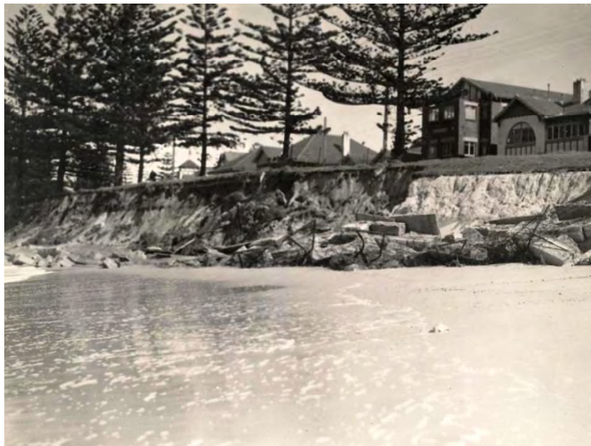
Figure 4.5 North Steyne Seawall Collapsed in front of Pacific Street (25/05/1943)
