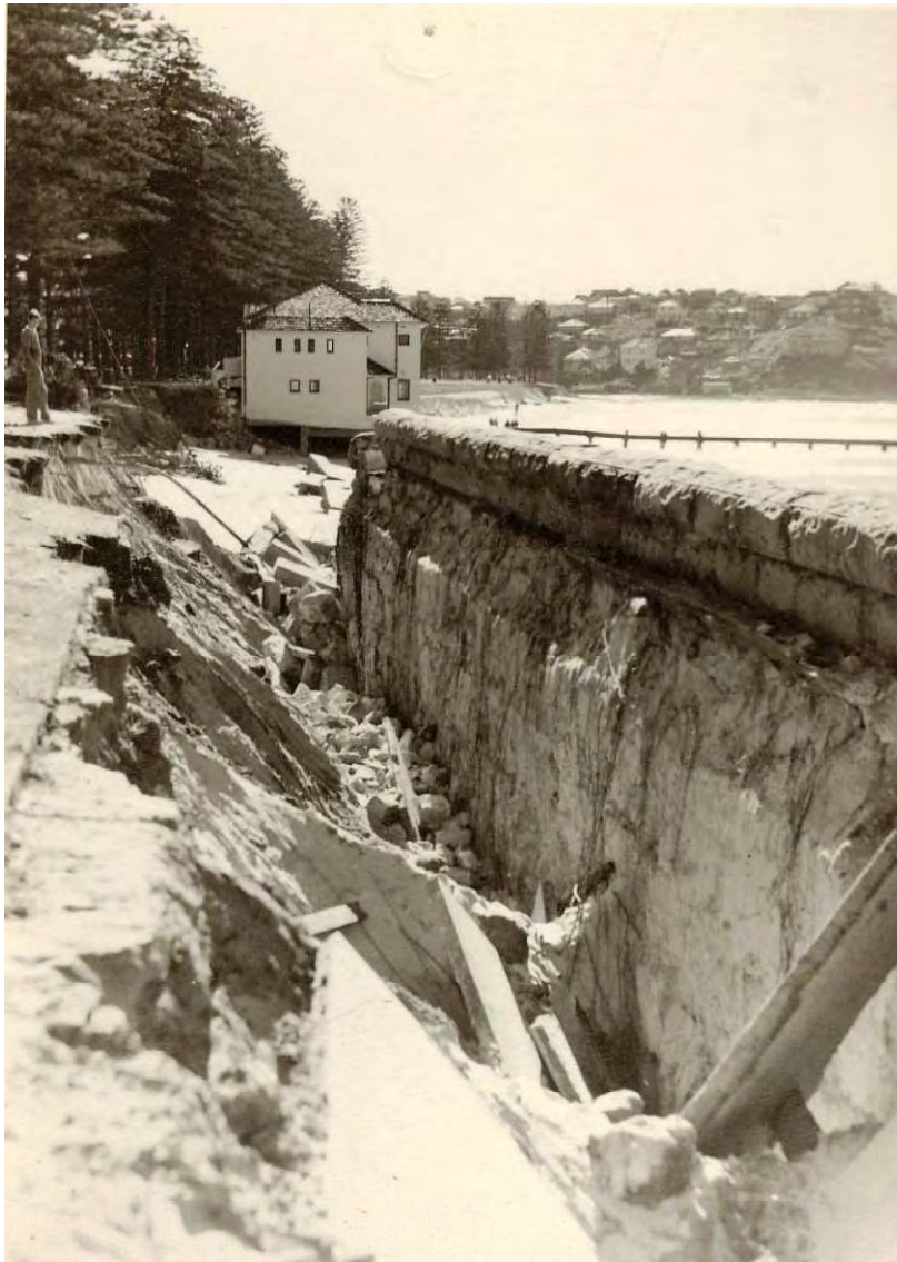
Figure 5.4 North Steyne Collapsed Seawall 27/06/1950
